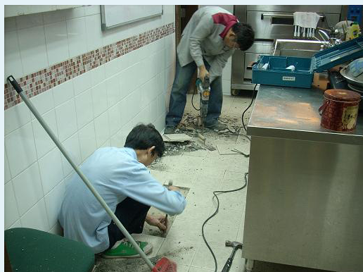
To repair the floor tiles at the CFAE Teaching Kitchen on the 2nd floor of Block A Caritas House
